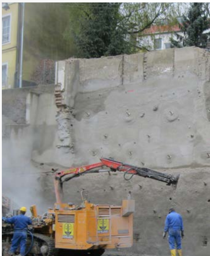
Installation de clous DURGLASS®
