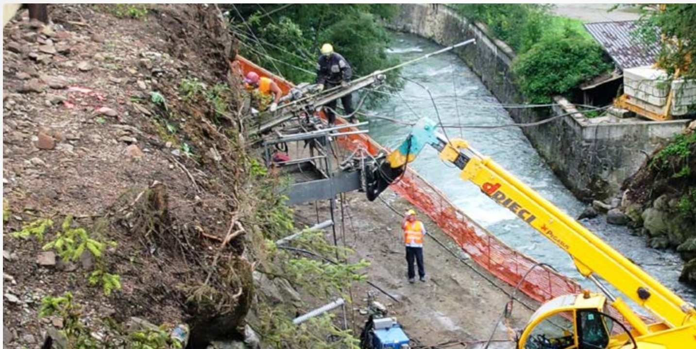
Installation de tirants DURGLASS®
